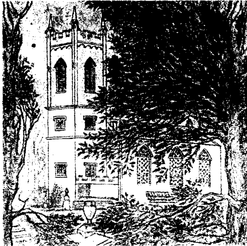
Figure 2. The Abbey Church: An old drawing showing the pinnacles on the tower.
